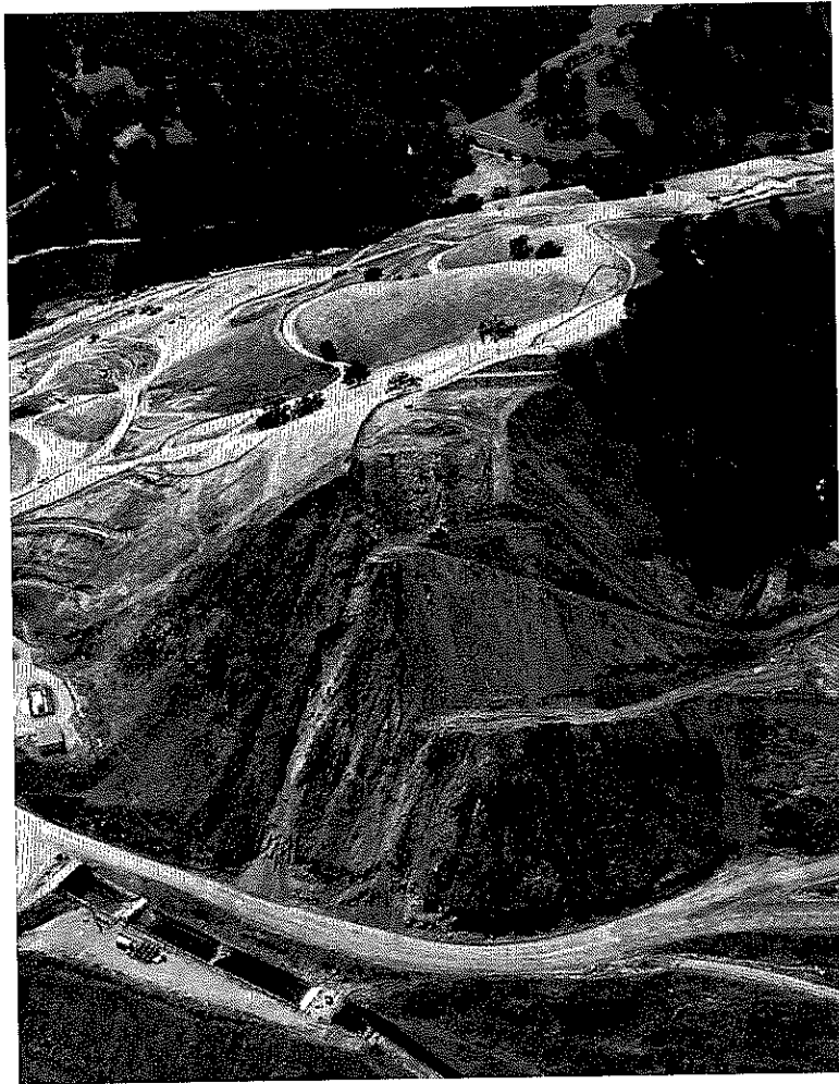
Photo 1 – Left Abutment Excavation
