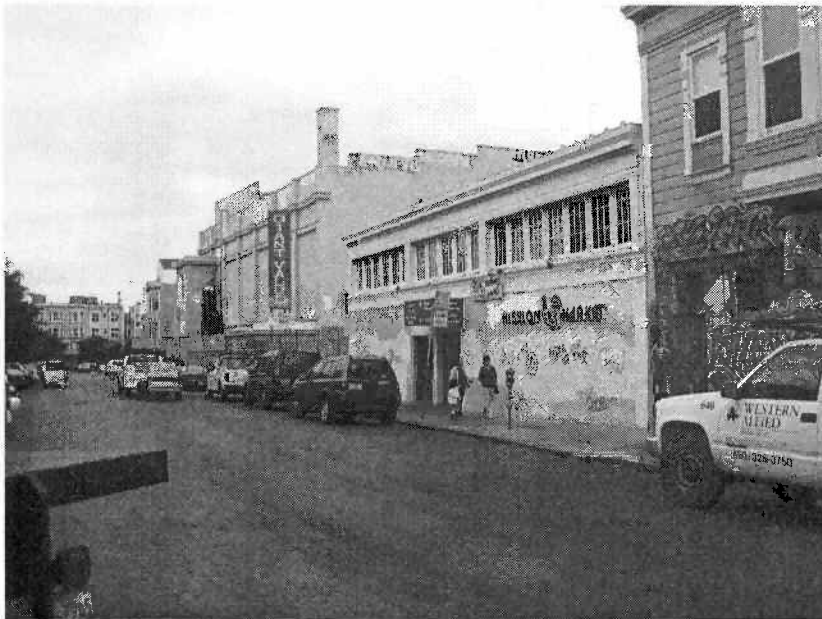
View of the Bartlett Street adjacent to the 2550-2558 Mission Street project site
