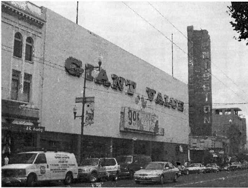
View of the Mission Street frontage of the 2550-2558 Mission Street project site
