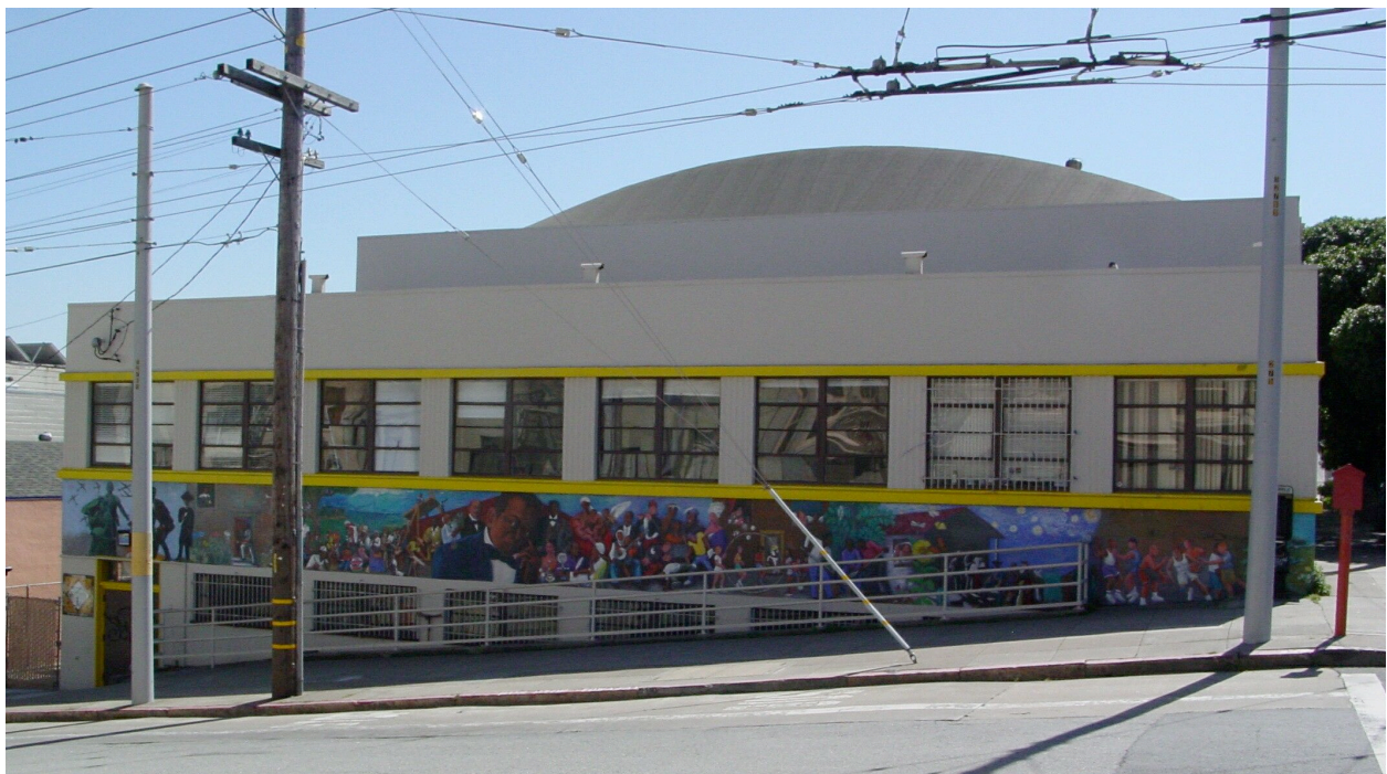
Fig.8 – North Elevation from Sutter Street
