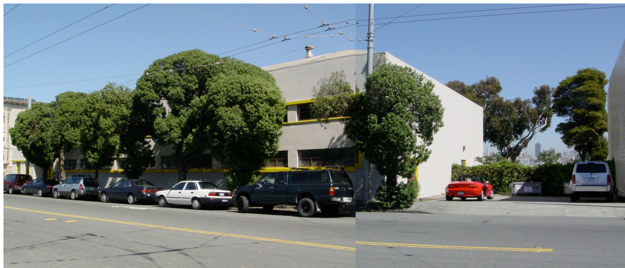
Fig.5 – West Elevation with South Yard at right
