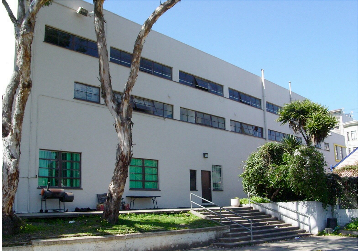
Fig.9 – East (rear) Elevation from Rear Yard
