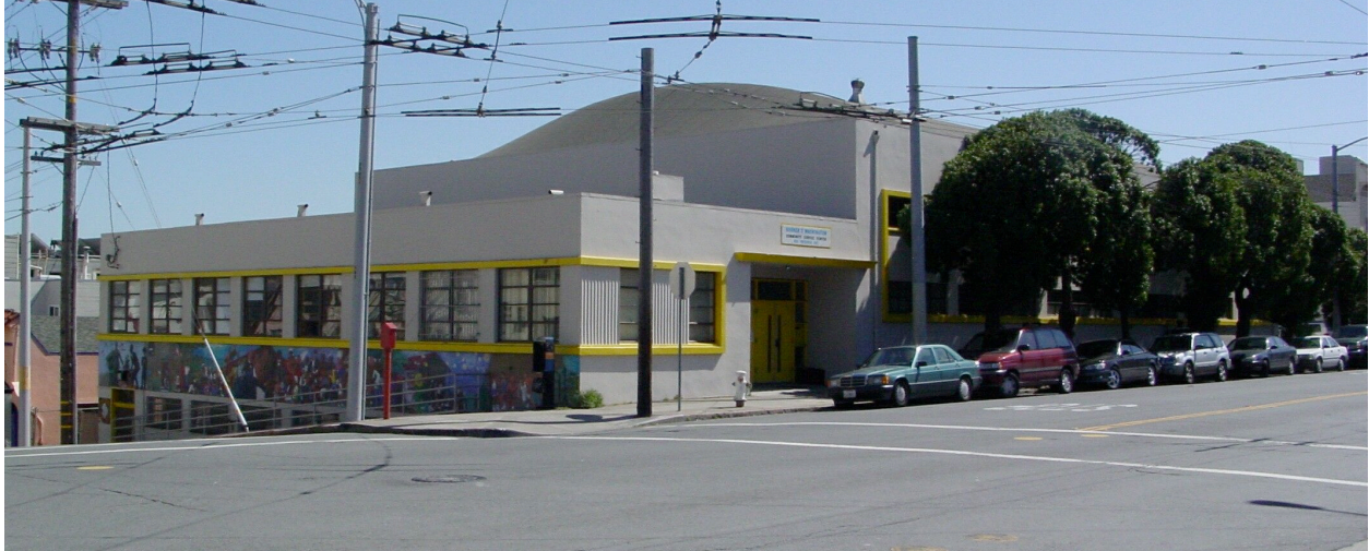
Fig.6 – BTW viewed from corner of Presidio (at right) and Sutter (at left)
