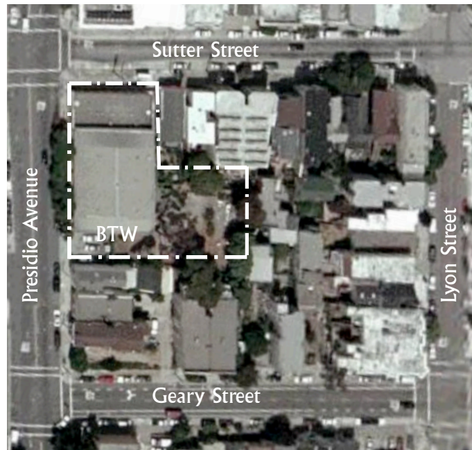
Fig.1 – Aerial View of BTW Building and Site (north is up)
