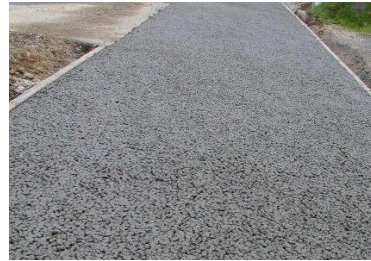
Porous concrete for permeable parking area
