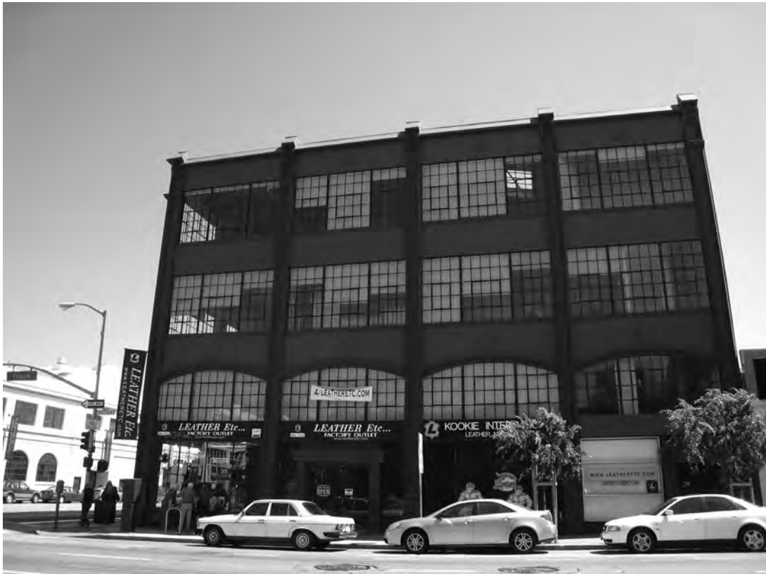
Commercial building at Eighth and Folsom Streets
