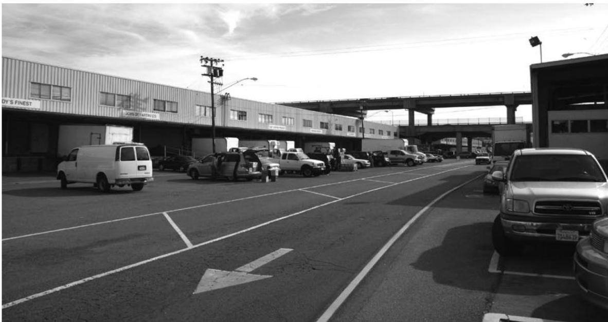
B. View Looking East at Existing Building L
