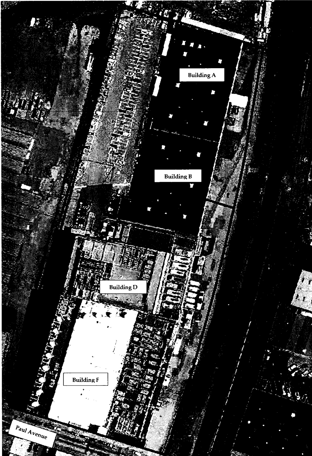
Figure 2 - Aerial Photo of Project Site
