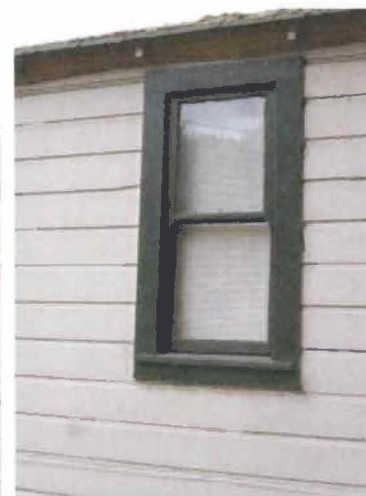
Figure 53. Detail of wood-sash window on south façade Source: Page & Turnbull, 2013
