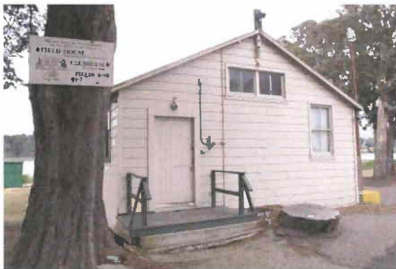
Figure 39. Southeast façade. Source: Page & Turnbull, 2013
