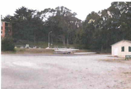
Figure 20. Edge slope at west end of the PRGC grounds. Source: Page & Turnbull, 2013
