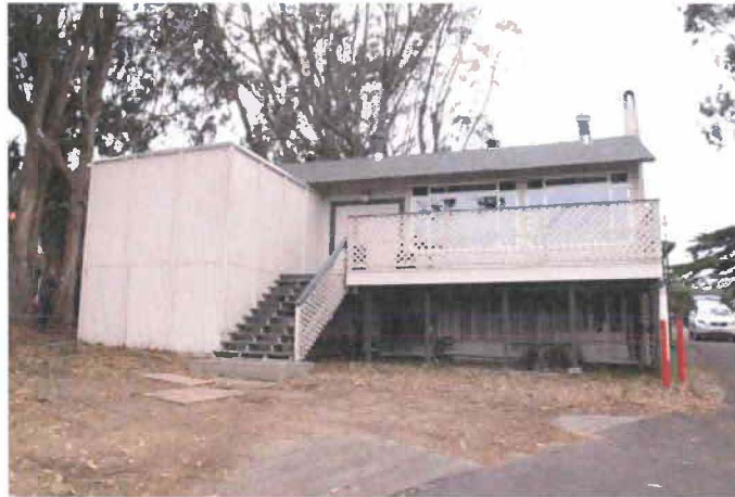
Figure 64. East façade. Source: Page & Turnbull, 2013
