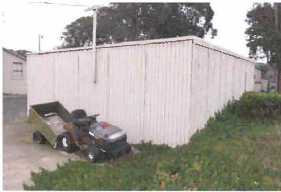
Figure 47. West facade Source: Page & Turnbull, 2013
