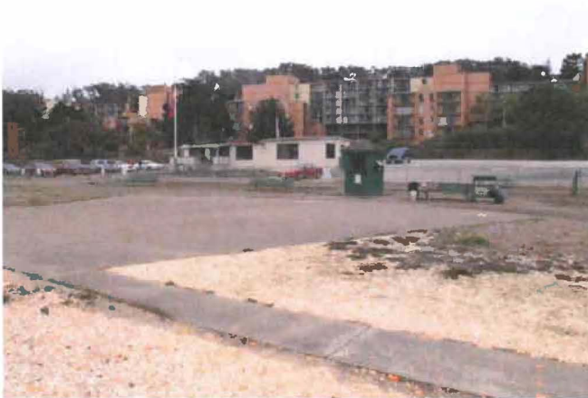
Figure 15. Concrete apron on Field 4 Source: Page & Turnbull, 2013
