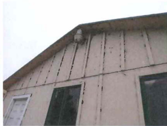
Figure 32. Detail of gable on southeast façade. Source: Page & Turnbull, 2013
