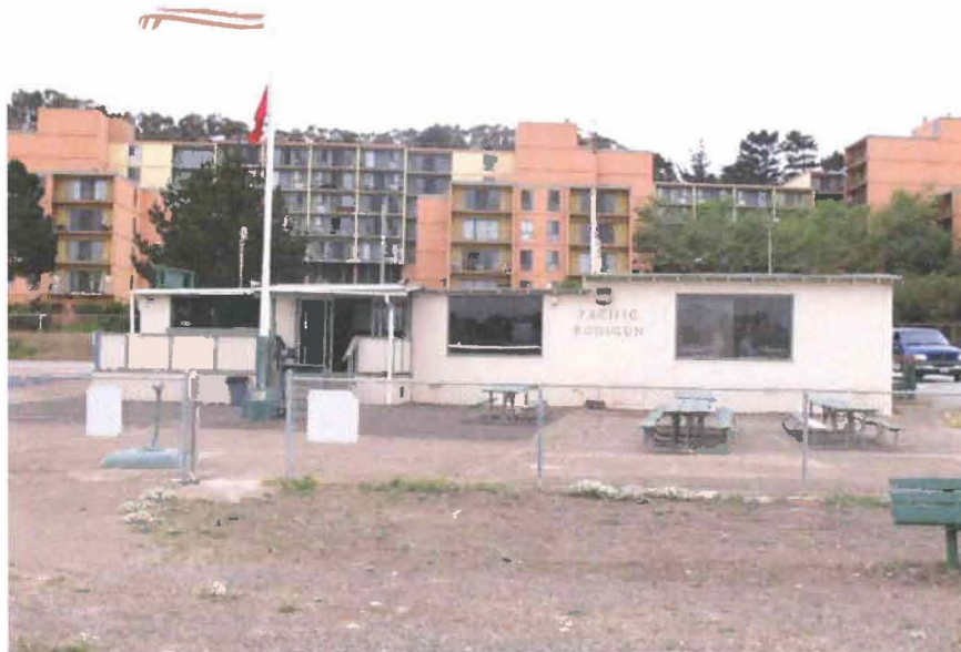
Figure 22. Northeast façade of the Club house, viewed facing southwest Source: Page & Turnbull, 2013
