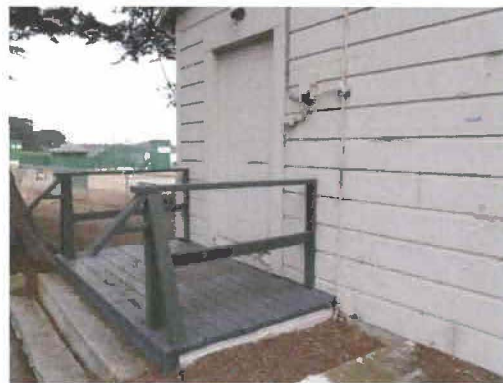
Figure 40. Detail of landing on southeast façade. Source: Page & Turnbull, 2013
