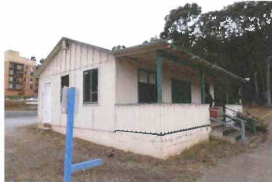
Figure 29. Southeast and northeast facades, viewed facing west.
