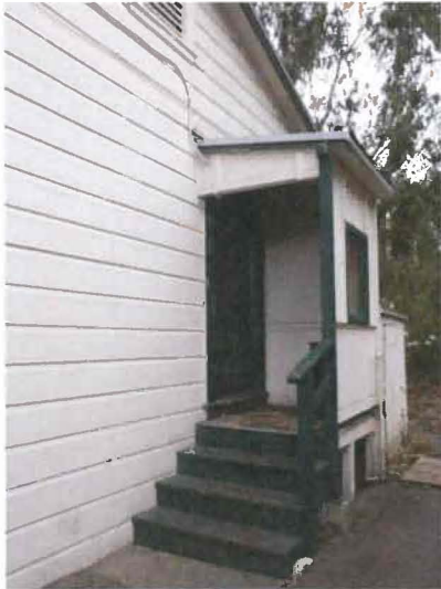
Figure 61. Detail of portico on west façade. Source: Page & Turnbull, 2013
