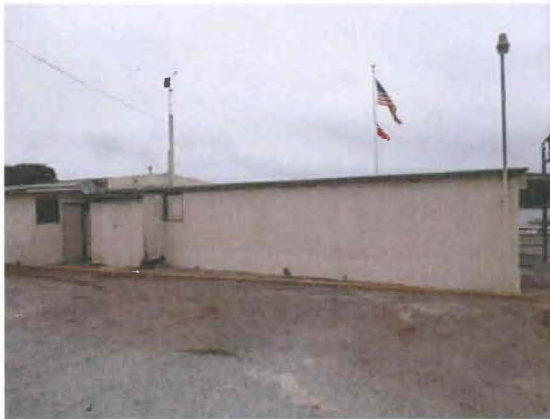
Figure 25. East end of southwest façade, viewed facing northeast. Source: Page & Turnbull, 2013
