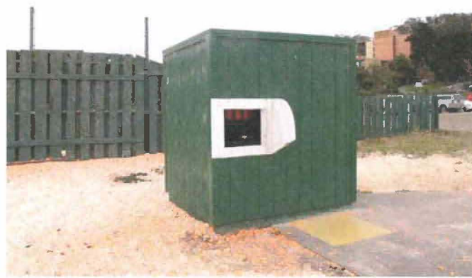
Figure 69. Field 4 low house. Source: Page & Turnbull, 2013
