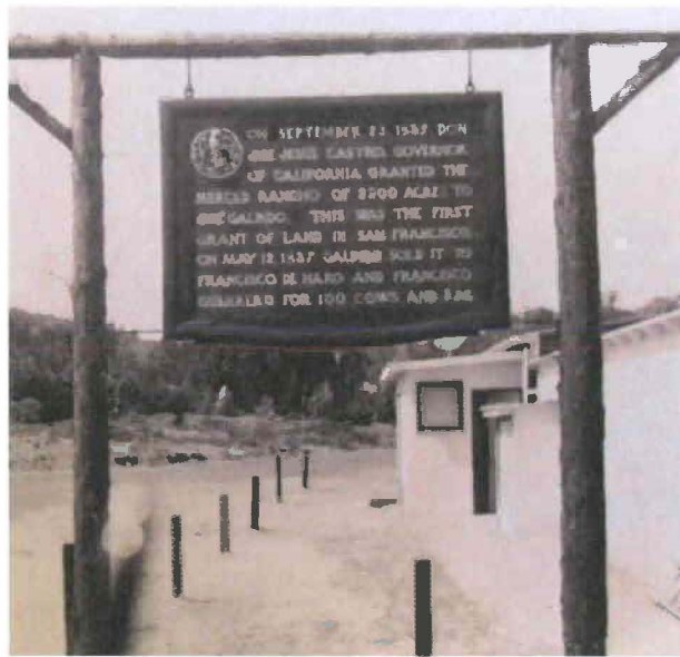
Figure 113. Historical wayside sign with original holder, to the rear of the Field house, c. 1950. Source: Pacific Rod and Gun Club
