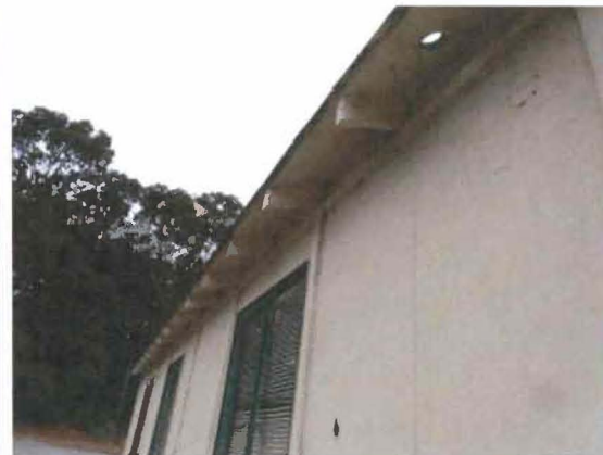
Figure 34. Rafter tails under eaves on southwest façade. Source: Page & Turnbull, 2013
