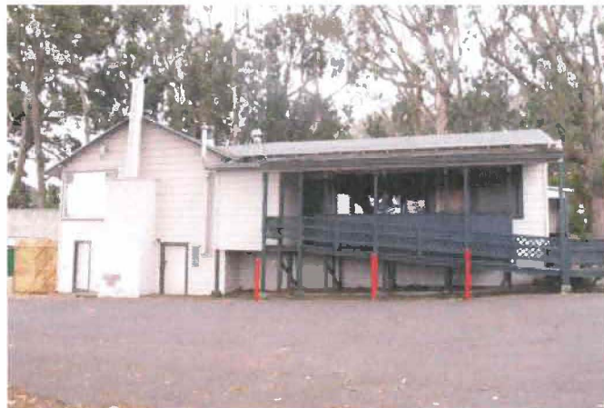
Figure 55. East and north facades of the Club House, viewed facing southwest. Source: Page & Turnbull, 2013
