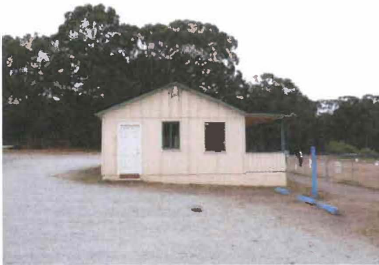
Figure 31. Southeast façade, viewed facing northwest. Source: Page & Turnbull, 2013
