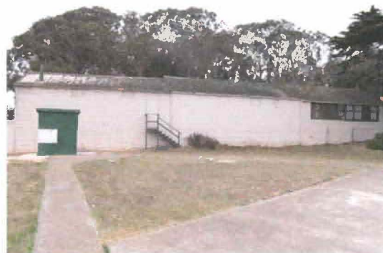
Figure 44. Northwest façade. Source: Page & Turnbull, 2013
