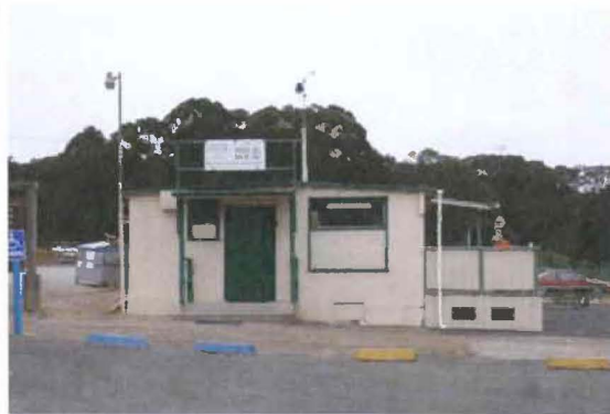
Figure 24. Southeast façade, viewed facing northwest. Source: Page & Turnbull, 2013
