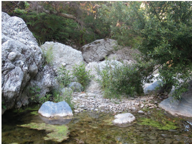
2a - Existing view of Feature 9 Tailwater Weir, looking downstream.
