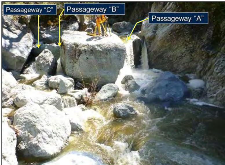
Flow plunging over Feature 10 Passageways A, B, and C at 36.0 cfs.
