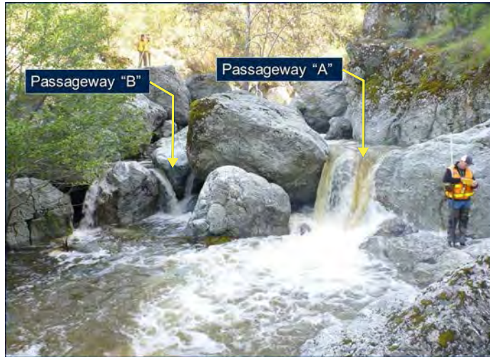
Flow plunging over Feature 9 Passageways A and B at 38.5 cfs.
