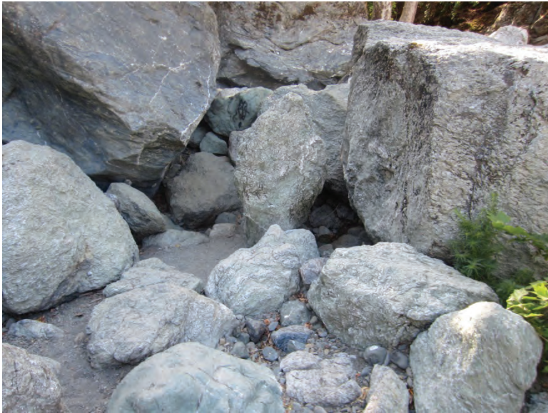
2a. Existing view of Feature 10 Step Weir B site, looking upstream.
