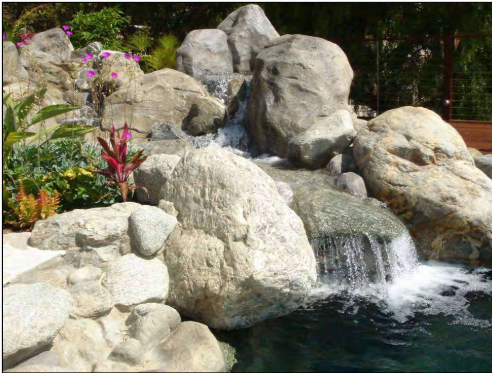
An example of an artificial boulder water feature formed entirely of concrete.
