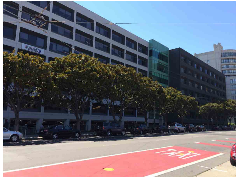
17. View north of the west side of Harrison Street from Third Street
