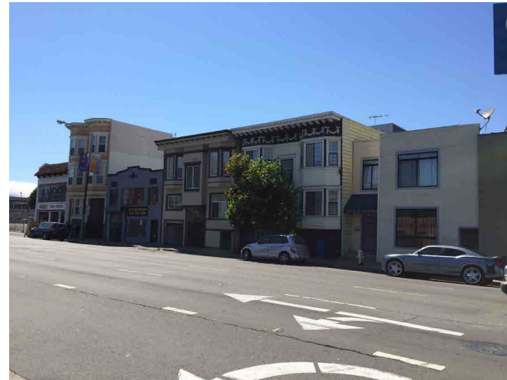
14. View west of the north side of Harrison Street between Fifth and Sixth Streets
