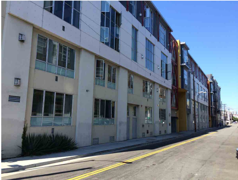
18. View east of the north side of Bluxome Street from Sixth Street
