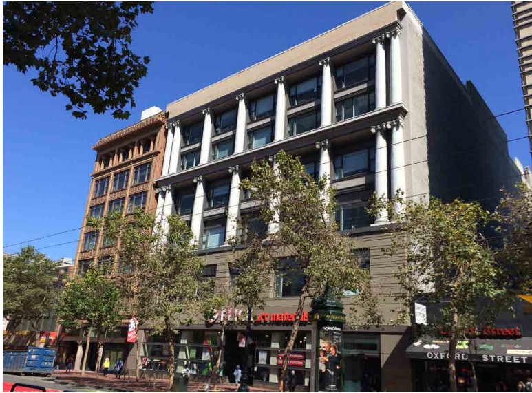
30. View of buildings on the south side of Market Street between Fifth and Sixth Streets located in the Market Street Theater and Loft Historic District
