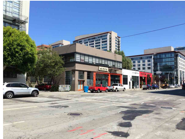
21. View south of the east side of Fourth Street from Bluxome Street
