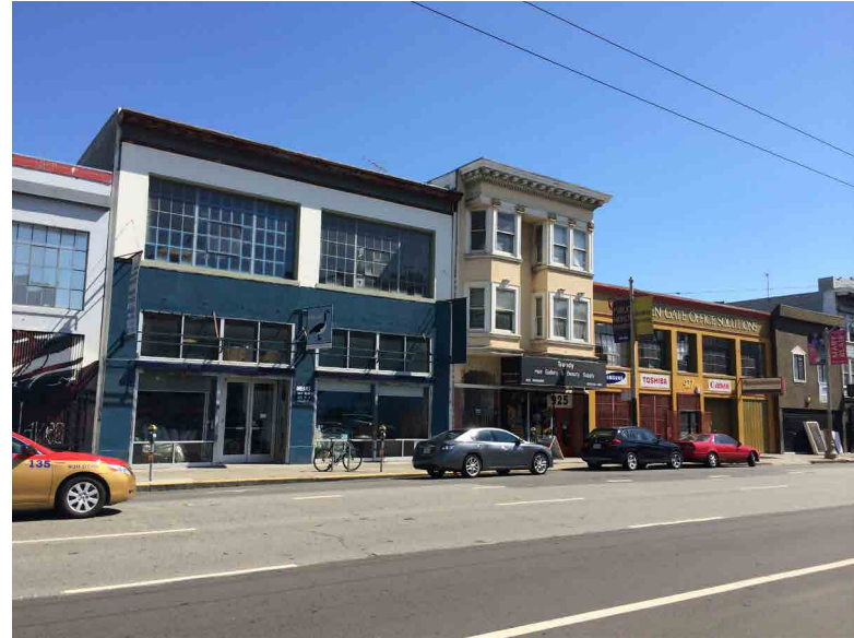
16. View west of the south side of Howard Street between Fifth and Sixth Streets
