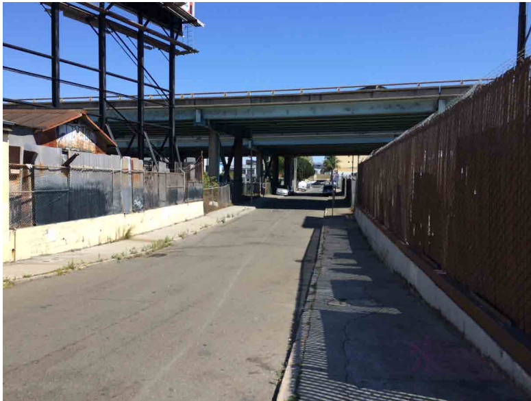
28. View south of Morris Street from Harrison Street
