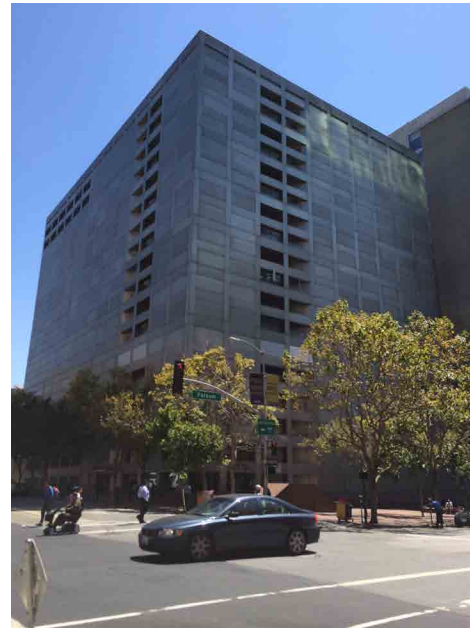
12. View of the southwest corner at Folsom and Second Streets
