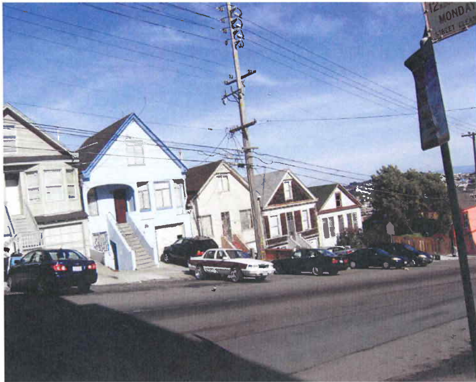
1) View of the adjacent properties to the west.
