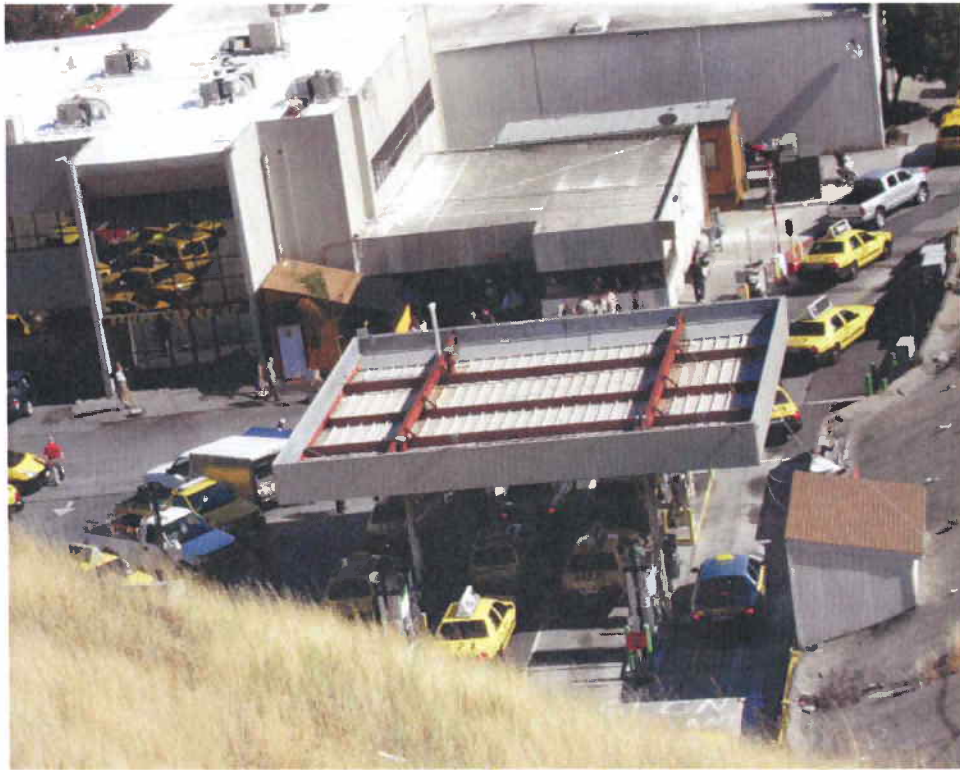
1) View of the adjacent property to the south.
