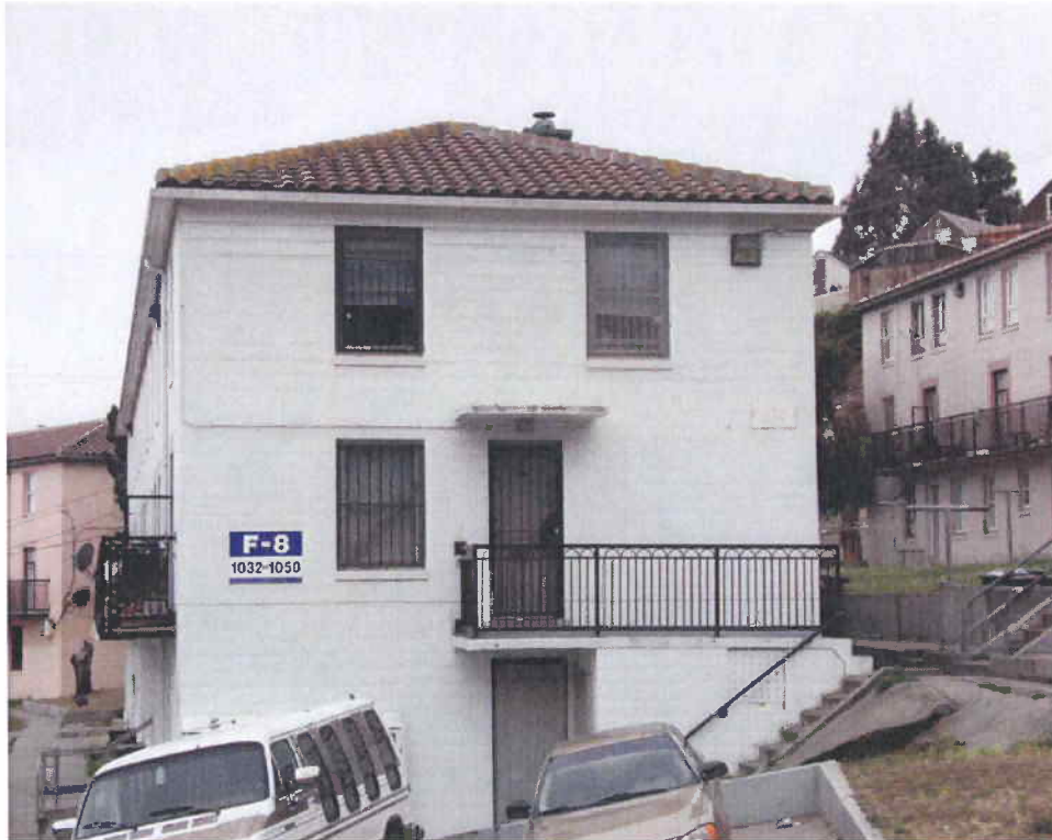
2) View of the Site buildings looking west.
