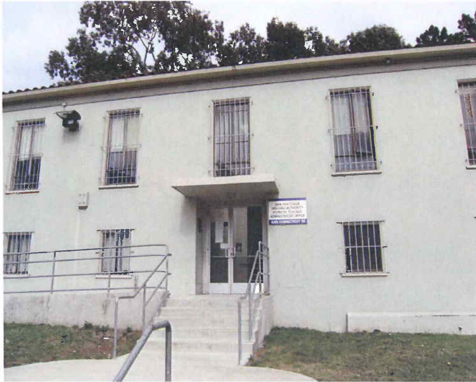
1) View of Potrero Terrace administrative office.
