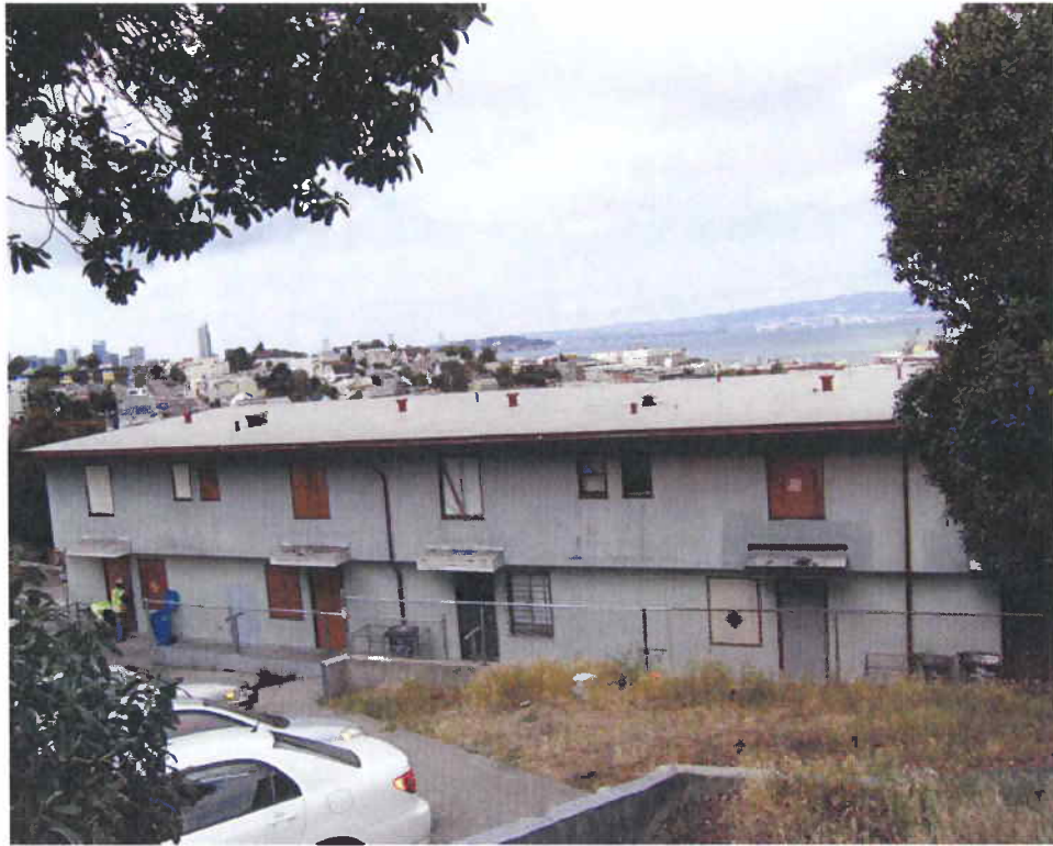
1) View of rear elevation of building, looking northeast.
