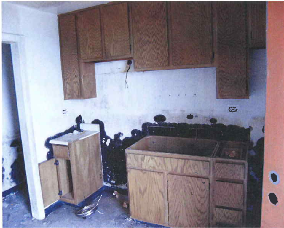
1) Interior view of a typical vacant unit.
