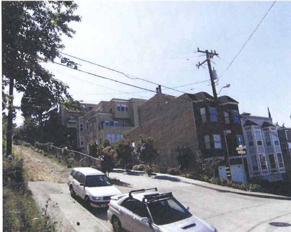
2) View of the adjacent properties to the north.
