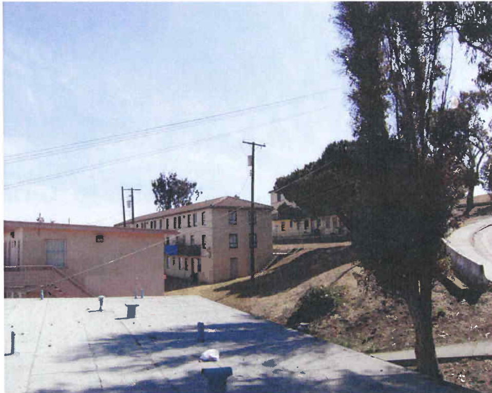
2) View of the Site building looking south.
