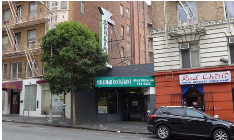
Figure 24. The west elevation of 530-532 Jones Street.
