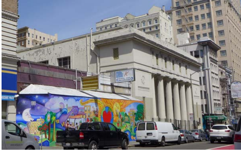
Figure 6. The west elevation partially seen from O'Farrell Street.
