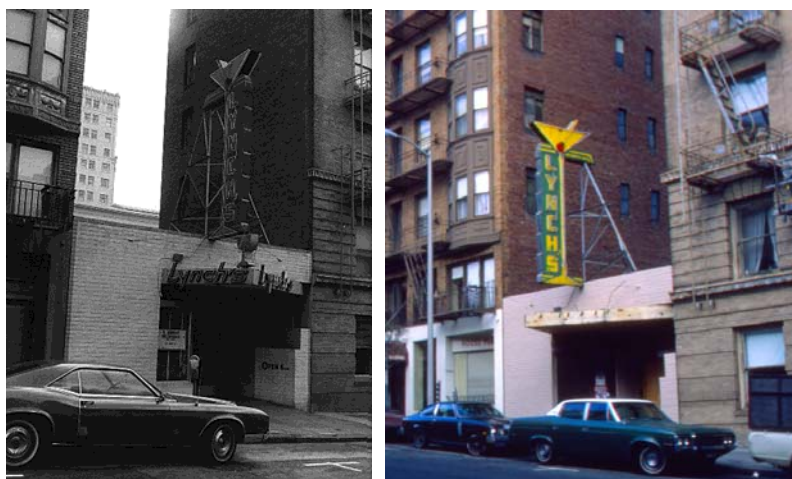
Figures 36 and 37. 530-532 Jones Street in 1976 (left) and in 1985 (right). 72
