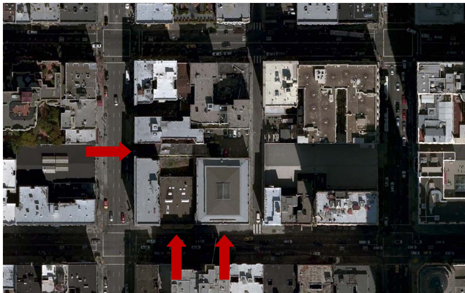
Figure 1. Aerial view of 530-532 Jones Street (top left), 474-480 O'Farrell Street (bottom left), and 450 O'Farrell Street (bottom right), marked by red arrows (Bing Maps, accessed on April 13, 2015).
