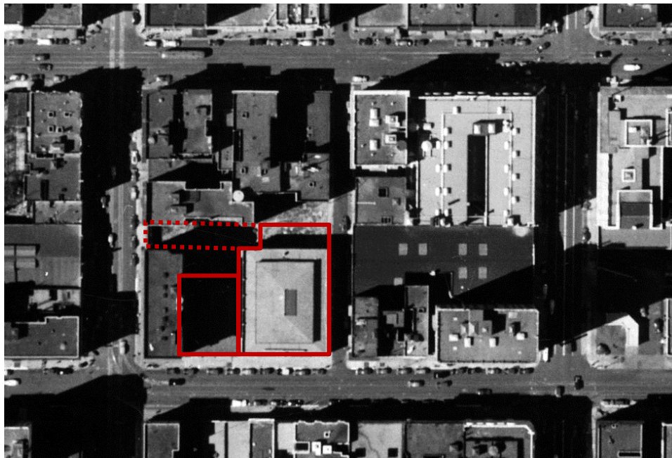
Figure 30. 1938 aerial photograph of the block from the David Rumsey Historical Map Collection.
