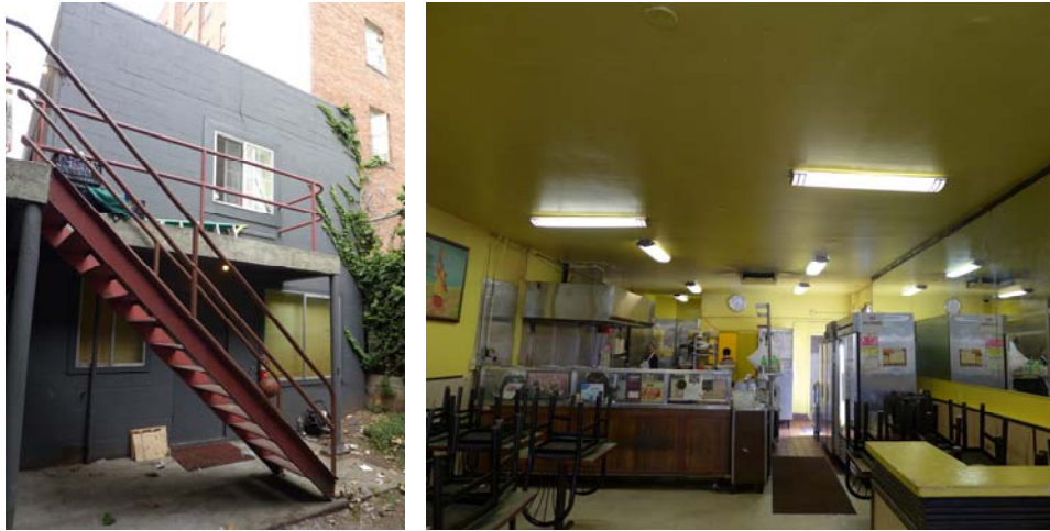
Figures 27 and 28. The east elevation (left) and the restaurant space (right).
