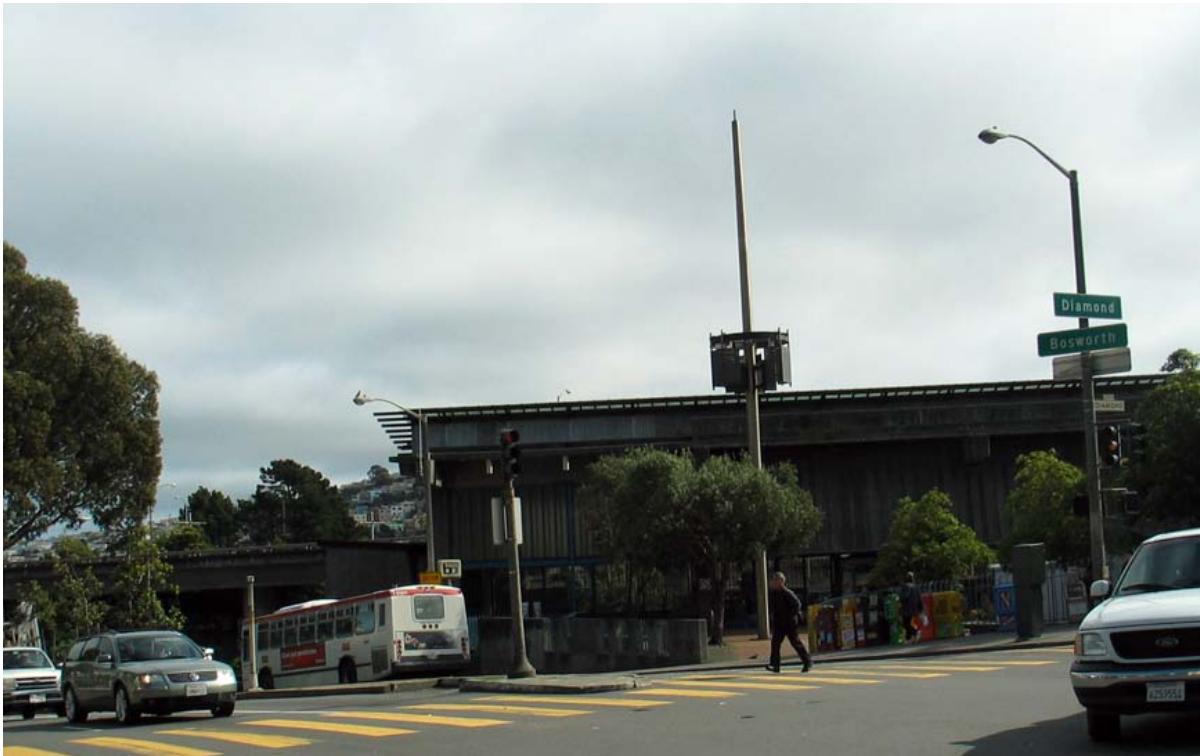
C. Glen Park BART Station. The Glen Park BART Station and the San Jose Avenue on- and off-ramps located south of Bosworth Street are the largest structural elements in the plan area, with solid concrete massing.
