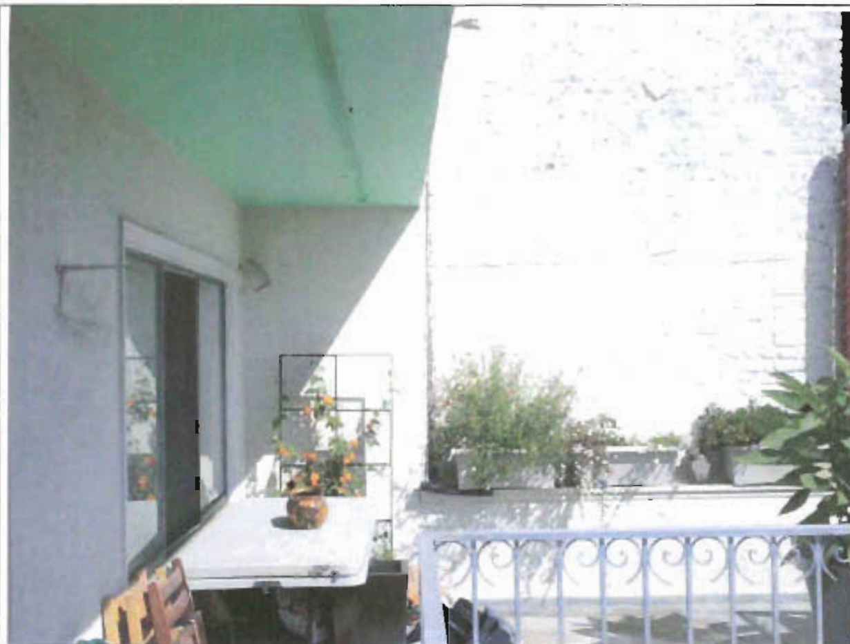
The rear terrace of 55 Dolores, Unit #1 currently enjoys the privacy and security afforded by the wall. Loss of the wall will "open up" the entire side of the property, leaving it open to potential security problems.
