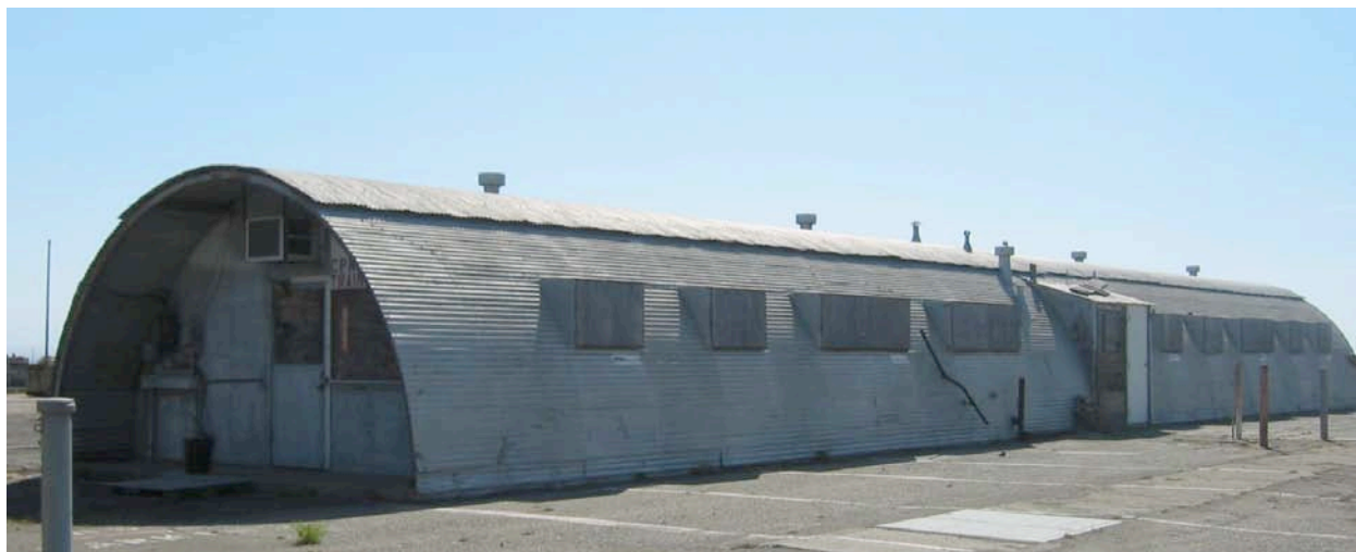
Figure 21. Building 367 is constructed of two Quonset huts placed end-to-end. This building type was used for housing along the south shore of Hunters Point during World War II. Photo: Circa, 2008.
