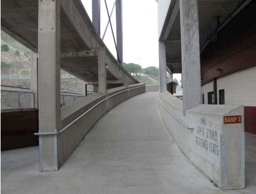
Figure 13. Original concourse (right) and later (c.1970) ramp (left), note differences in concrete. (Photo by Circa, 30 January 2010).
