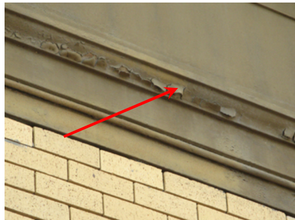
Figure 61. Delaminating paint. Source: Page & Turnbull, March 2010.
