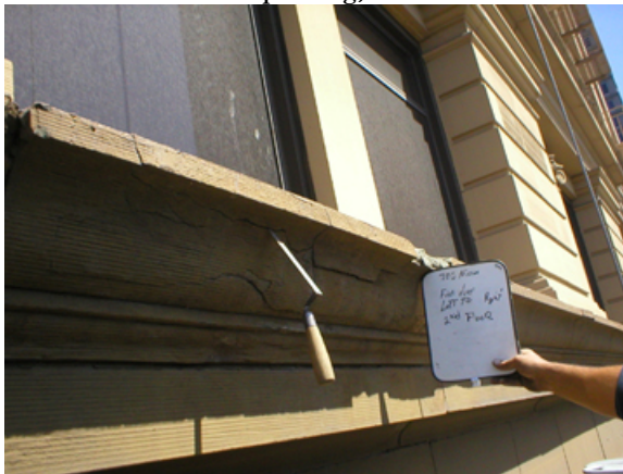
Figure 50. Cracking of sandstone. Source: Rainbow Waterproofing, 2006.
