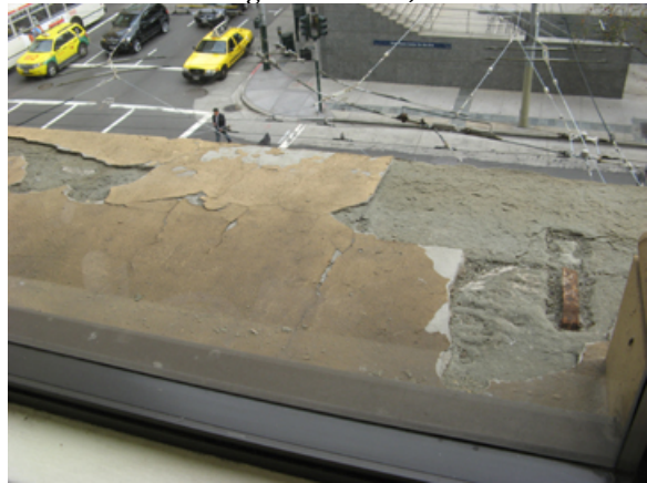
Figure 42. Exfoliation of crust. Source: Page & Turnbull, March 2010.
