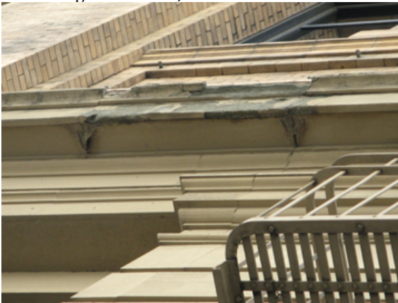
Figure 41. Spalling of sandstone at edge. Source: Page & Turnbull, March 2010.
