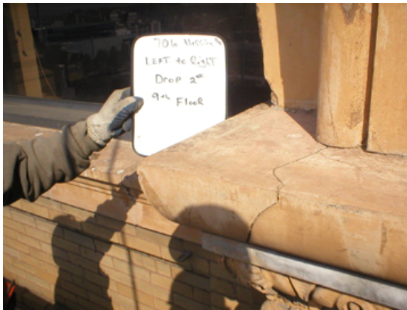
Figure 44. Cracking at cornice. Source: Rainbow Waterproofing, 2006.
