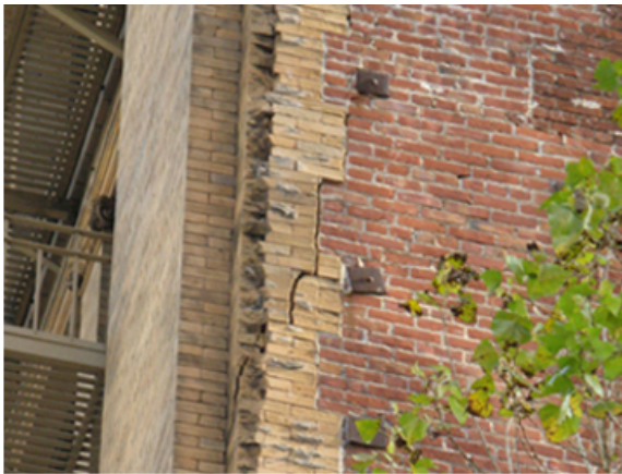
Figure 35. Cracking at terra cotta to brick interface. Source: Page & Turnbull, March 2010.
