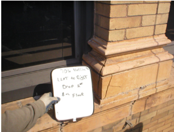
Figure 46. Cracking at column base. Source: Rainbow Waterproofing, 2006.
