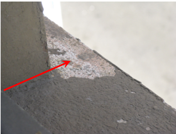
Figure 60. Corrosion of cast iron. Source: Page & Turnbull, March 2010.
