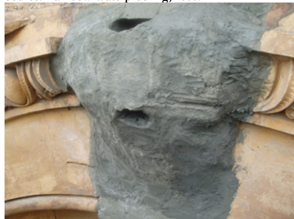
Figure 49. Removal of cracked and mortar patch of piece shown at left. Source: Rainbow Waterproofing, 2006.
