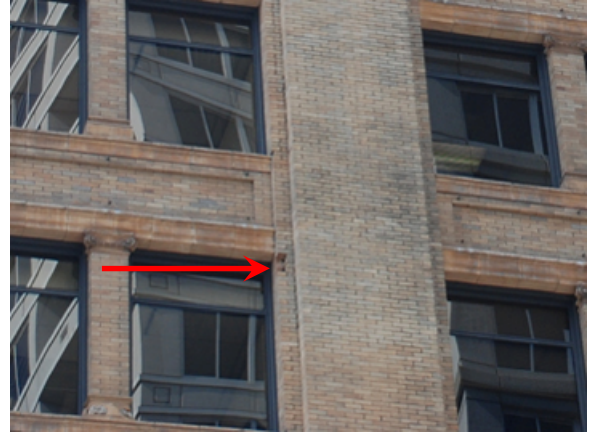
Figure 59. Missing brick. Source: Page & Turnbull, March 2010.
