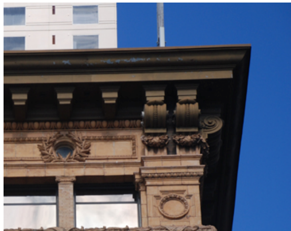
Figure 64. Area of exposed sheet metal with no paint. Source: Page & Turnbull, March 2010.
