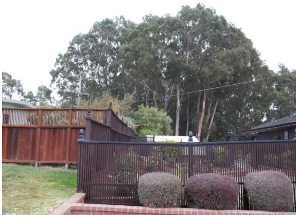
View 4: View to east from Ridgewood Drive to the construction zone in the SFPUC ROW
