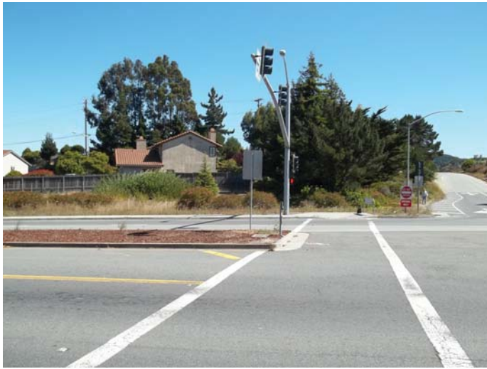
View 1: View to the south from San Bruno Avenue to the construction zone, adjacent to the I-280 off-ramp
