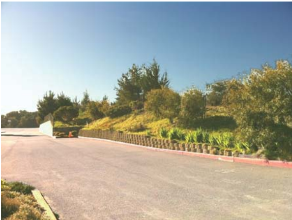
View 4: View to the south from San Bruno Chinese Church parking lot to the staging and spoils area
