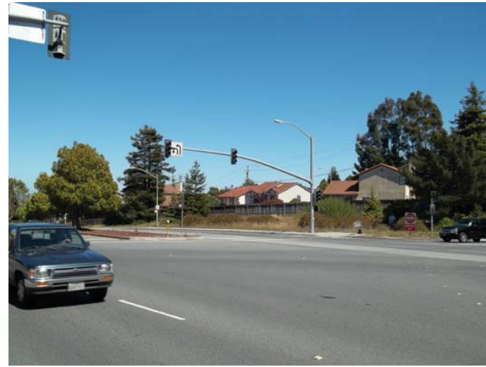
View 2: View to the southeast from San Bruno Avenue to the construction zone, adjacent to San Bruno Avenue
