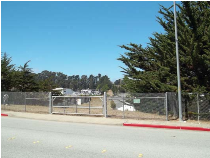
View 3: View to northwest from Collins Avenue to the construction zone in the SFPUC ROW
