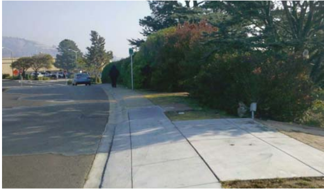
View 1: View to east from the driveway at 106 Arroyo Drive to the construction zone in the SFPUC ROW
