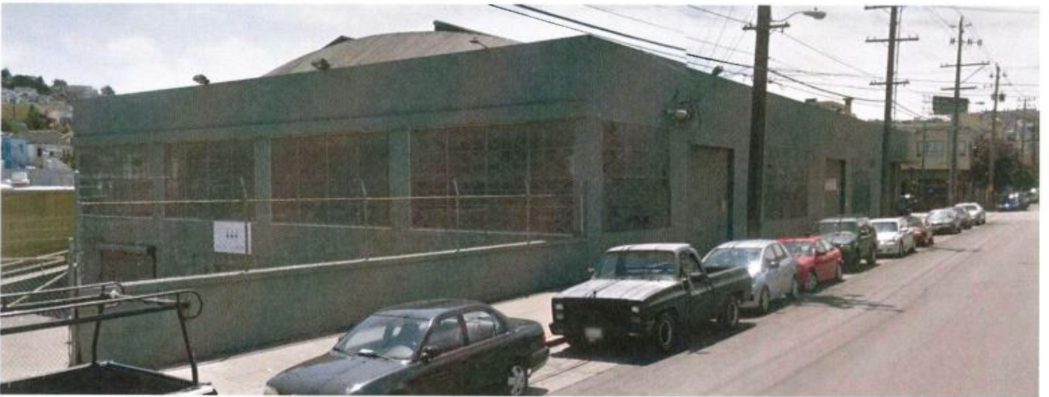
(Top photo) View of the subject property, at the southeast corner of 26 th St. and South Van Ness (Bottom photo) Rear of the subject property, from the down-sloping east end of the lot
