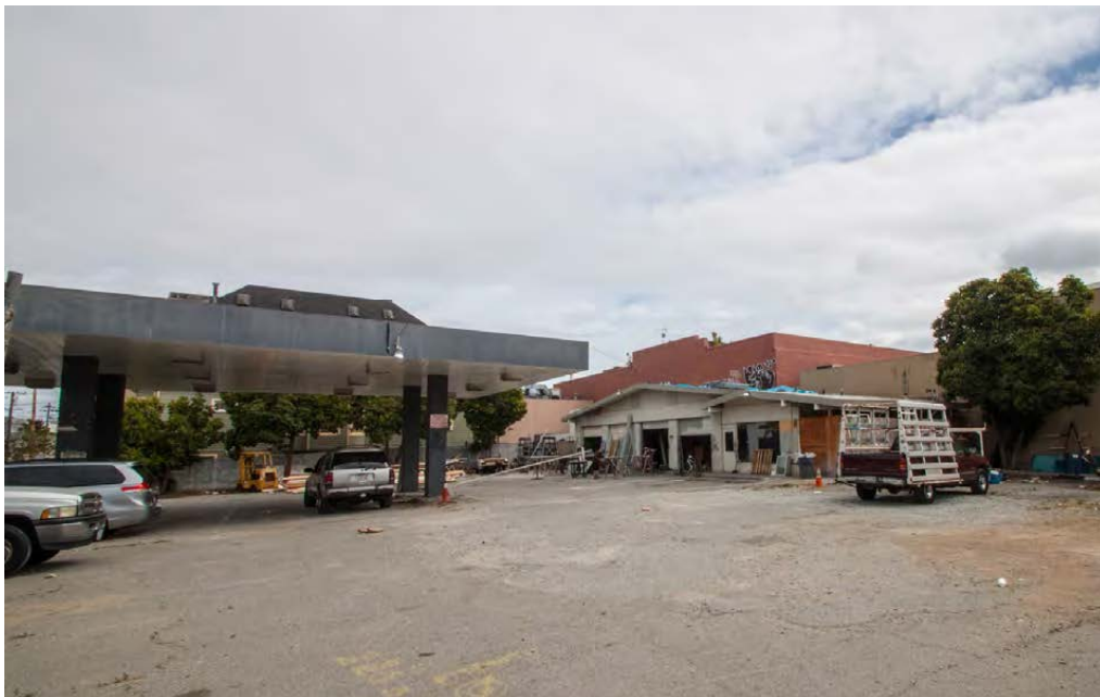
Figure 2. 793 South Van Ness Avenue (view looking northeast)
