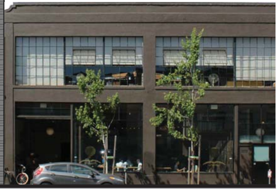
270 7TH STREET 2 LEVELS, APPROX. 30' TALL COMMERCIAL BUILDING W/ "SIGHTGLASS COFFEE"
