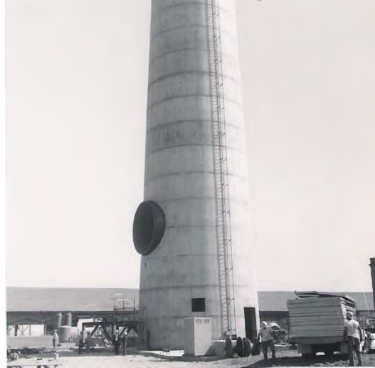
Figure 81: Boiler Stack without ducting (2 October 1964). Spreckels' East Wharf/Sugar Receiving building in the background. Source: Associate Capital.
