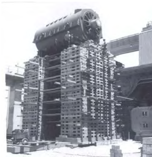
Figure 87: Unit 3 generator on blocks ready for placement (25 June 1965). Source: Associate Capital.
