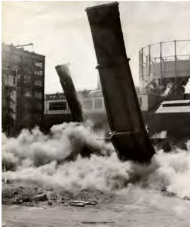
Figure 45: Demolition of two brick smokestacks at the Spreckels Sugar Refinery (9 August 1951). Sugar House at left. Source: San Francisco Public Library, Photo # AAC-7473.
