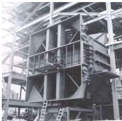
Figure 85: Unit 3 east air preheater (16 October 1964). Source: Associate Capital.
