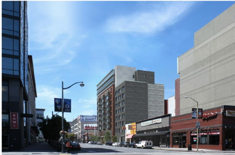
Photo 2: View looking towards Townsend Street from King Street.
